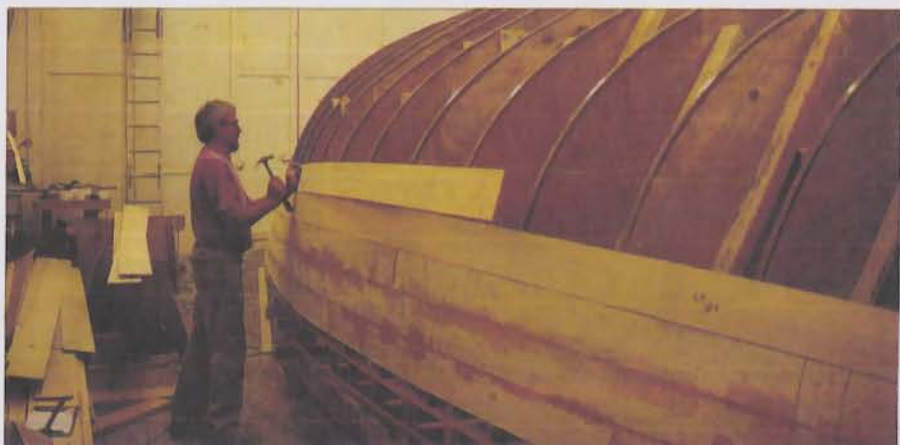
Covey Island's Terry Sundbo applies a first layer of planking on Sir Edmund's hull last September. Her construction is cold-molded cedar and Corecell foam.
