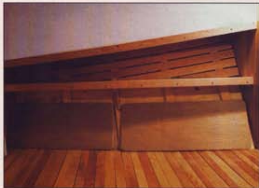
The base of this settee, formed by interlocking slats, pulls out to form a double guest bed supported by hinged legs.
